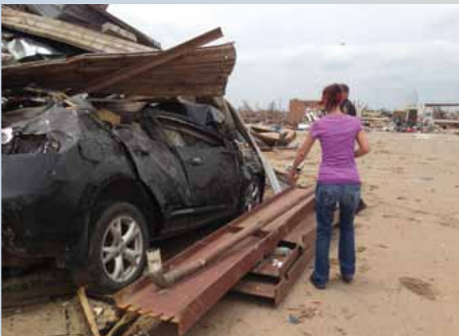
Oklahoma Farm Bureau Insurance Casualty Specialist Brooke Redinger inspects damage near Plaza Towers Elementary School in Moore. The school was located in one of the hardest hit areas during the May 20 tornado. OKFB Insurance employees were on the ground as soon as possible after this and other storms to help customers begin the recovery process.
